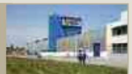
Hellenic Cables Livadia, Greece
